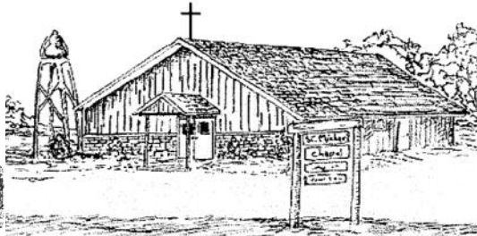
ST. MICHAEL STATION – Chute Pond
