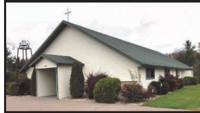
ST. MICHAEL STATION - Chute Pond
