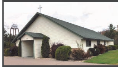
ST. MICHAEL STATION - Chute Pond
