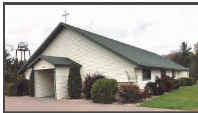
ST. MICHAEL CHAPEL- Chute Pond
